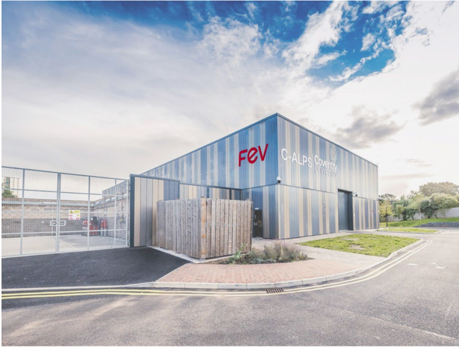
Caption: C-ALPS, one of UK's leading research facilities for hydrogen propulsion systems is jointly operated by FEV and Coventry University.
